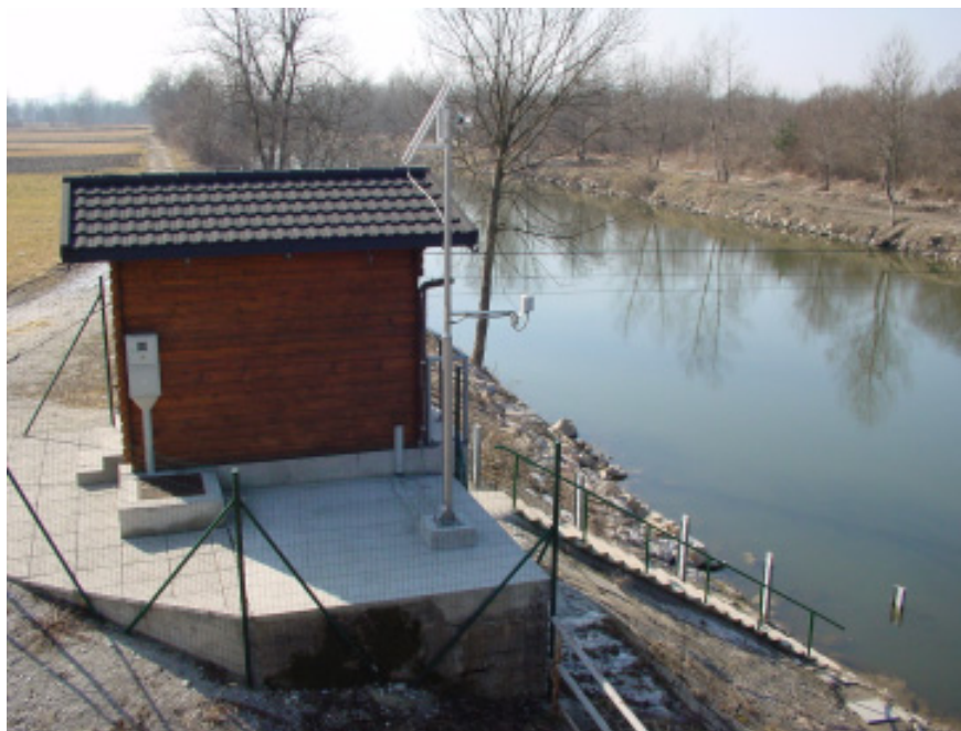
Slika 2. Vodometna postaja Šentjakob na Savi (foto: Arhiv ARSO) Figure 2. Gauging station Šentjakob on the Sava River (photo: Archives of ARSO)
